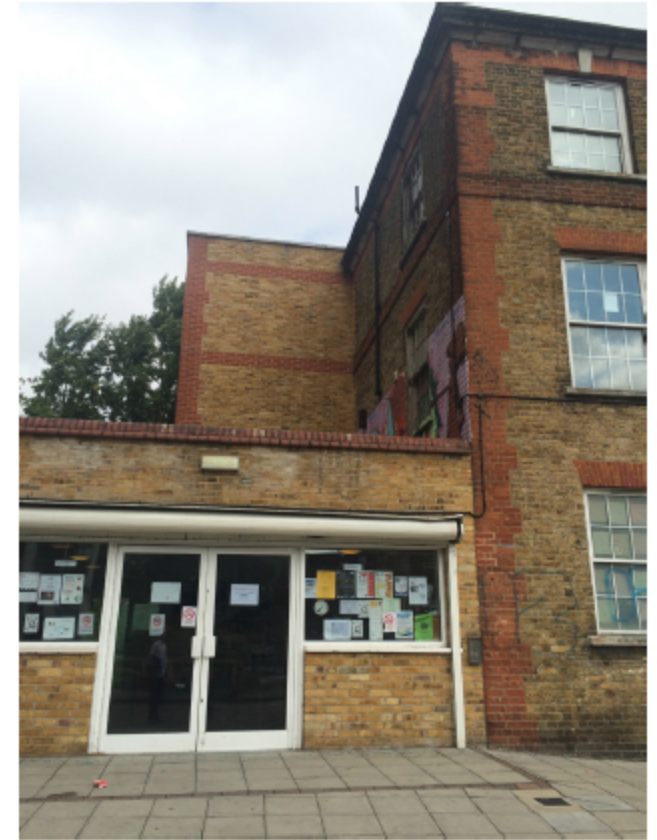
Existing entrance and single storey extension
